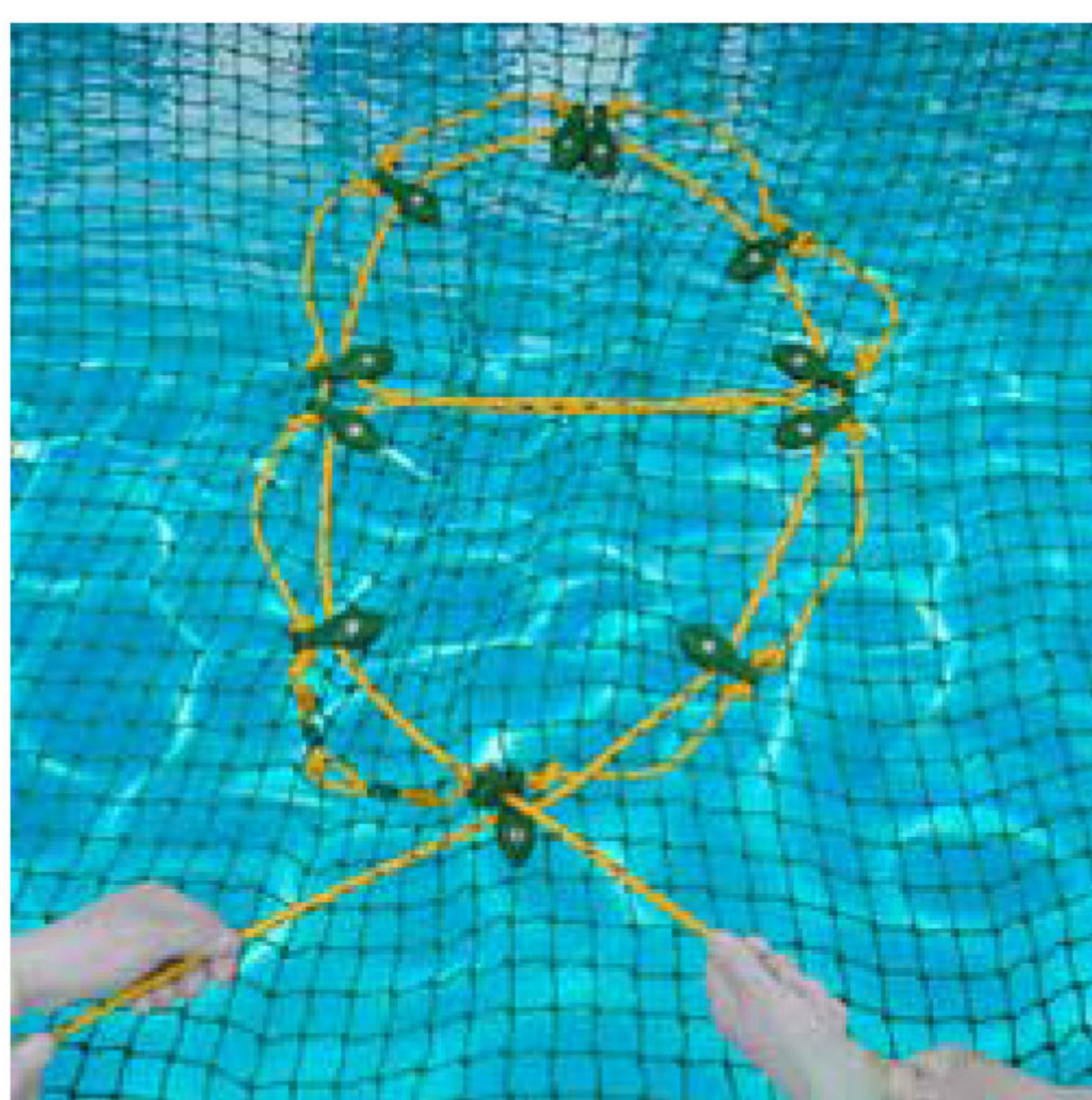
**A.** Begin tightening the net from one corner and move evenly around the pool to maintain uniform tension.
