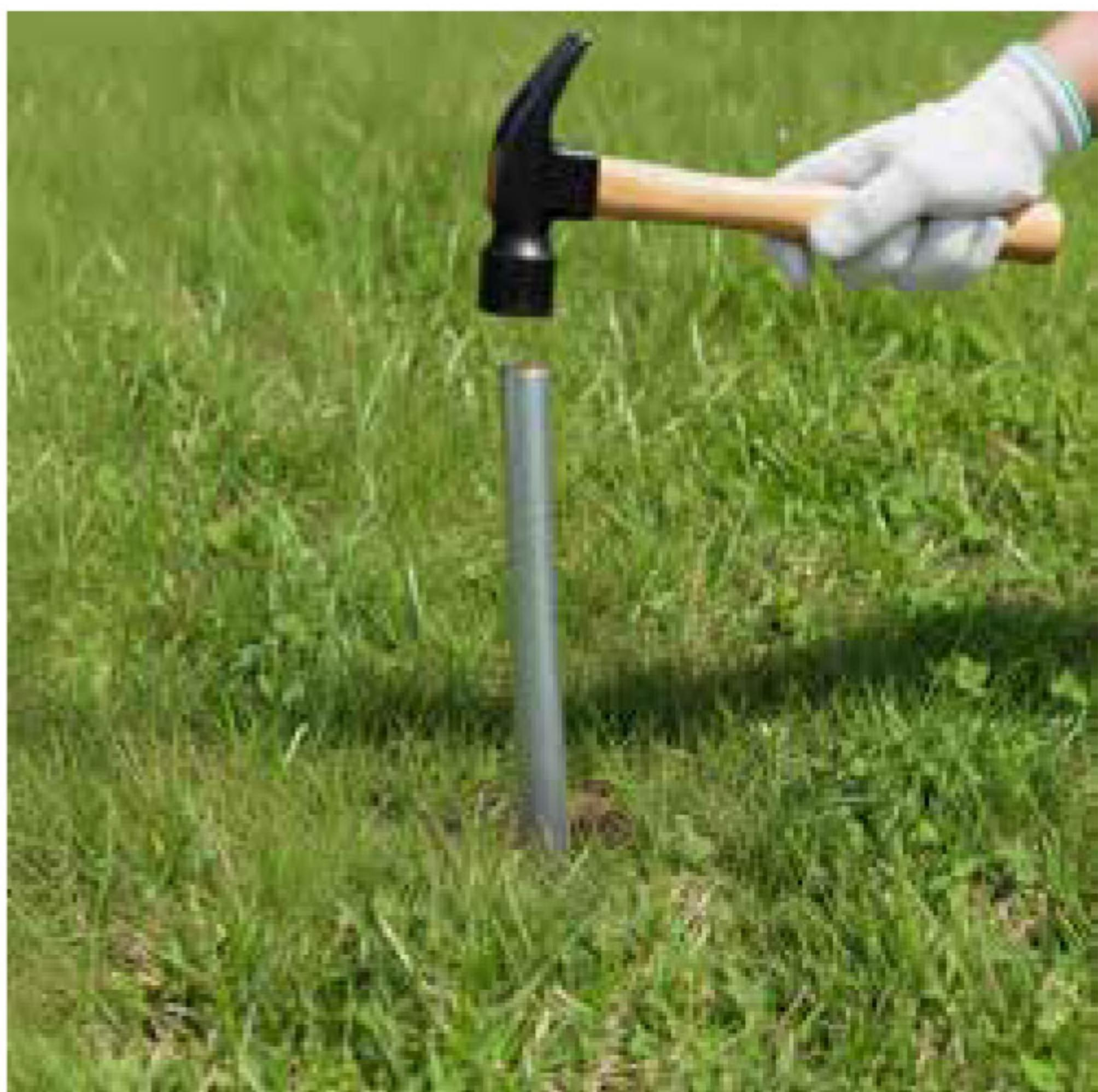
A. Fix the anchor into the hole using a mallet.
