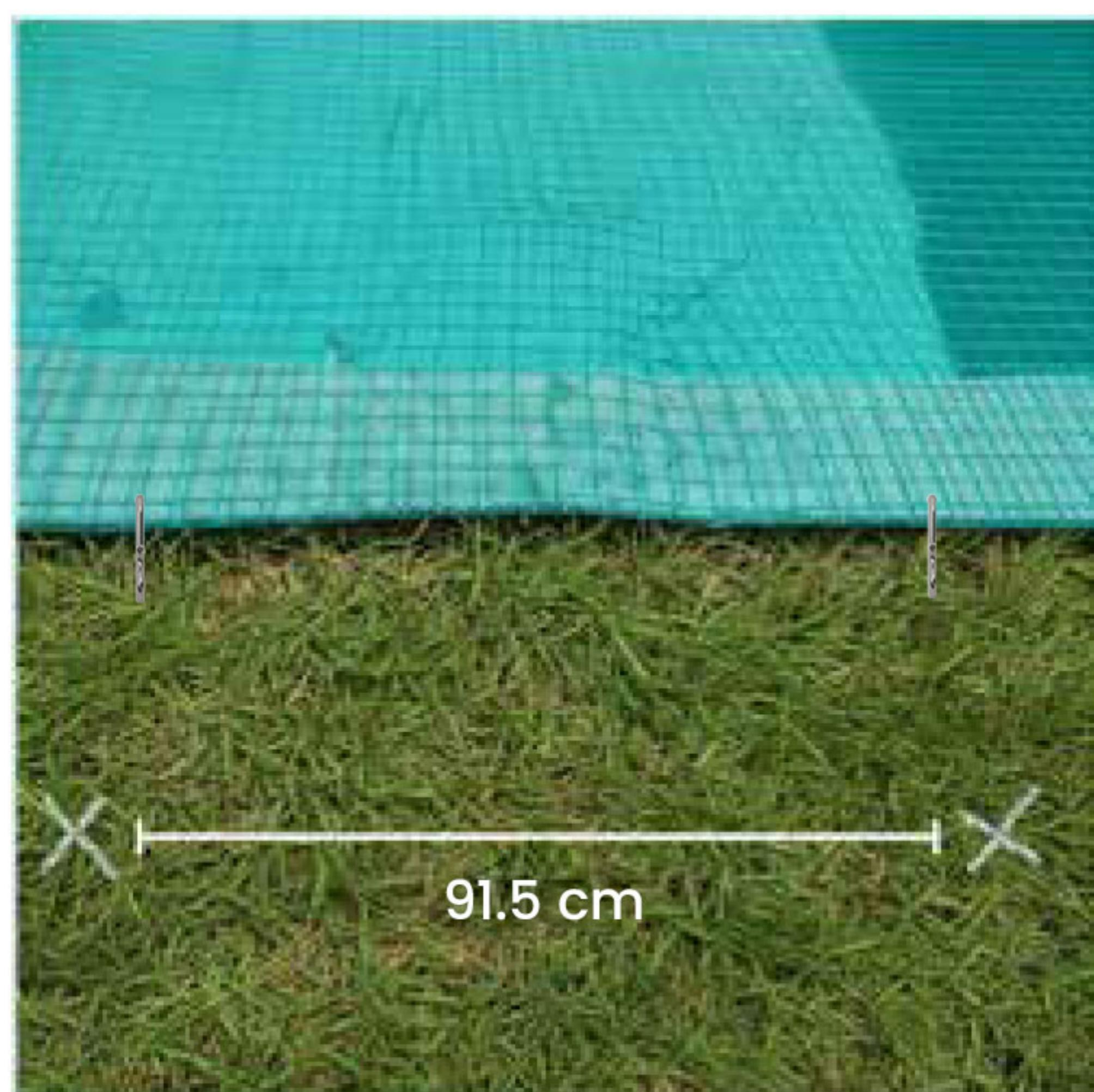
C. Align the marks in a straight, parallel line with prefixed SS clip on net.
